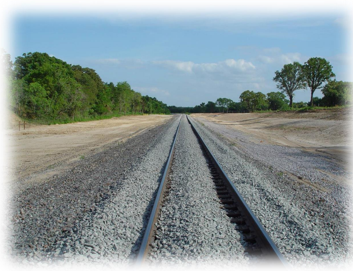
Cameron, Texas, post derailment
