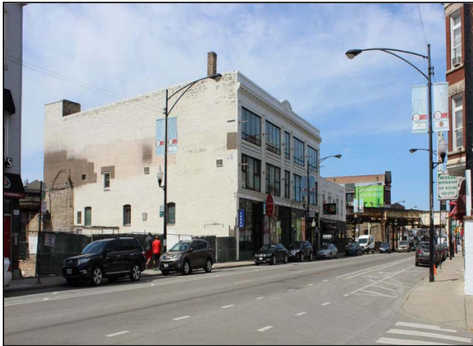
Existing Condition Photo
