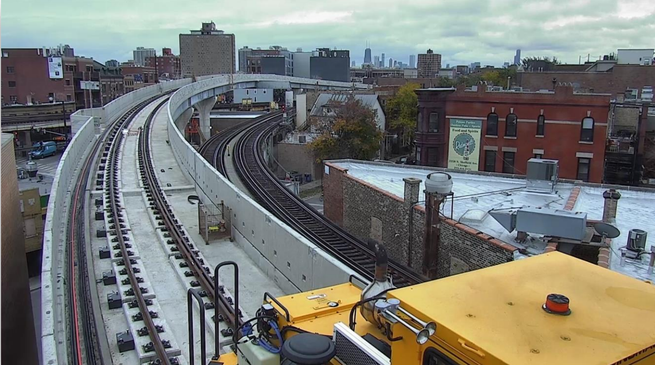
Bypass, facing east
